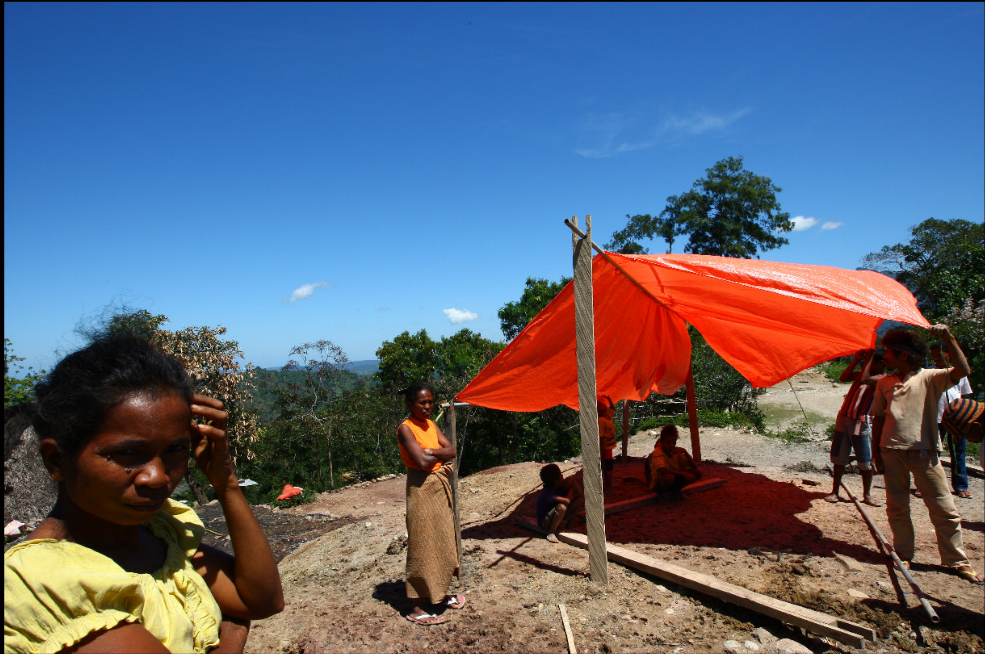
They are now busy building a temporary shelter for their family.
